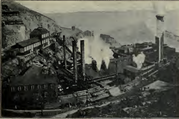
FIG. 33.—In these buildings metal is obtained from the ore that is mined in the mountain rocks far below the surface.
